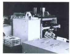
Folder/Feeder is positioned over the saddle-chain between the last hopper and the inspector unit. Shown here on a Harris Pacesetter, the unit can also be used with Macey and Sheridan inserter-stitchertrimmers.
